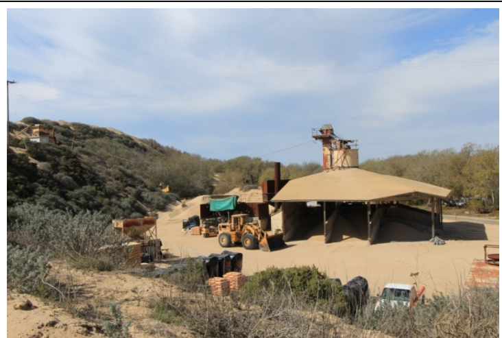
The Gordon Sand Company is a commercial sand mining operation that includes a sand screening and processing facility as well as an access road and sand collection pits. Access to the site is provided by a remnant unpaved road.
