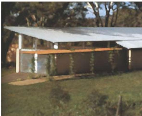
figure 3.6.1b: Simple, Low Pitch Shed Roof Forms - Glenn Murcutt.
